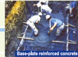
Base-plate reinforced concrete
