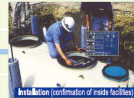
Installation (confirmation of inside facilities)
