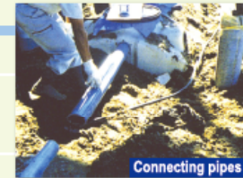
Connecting pipes
