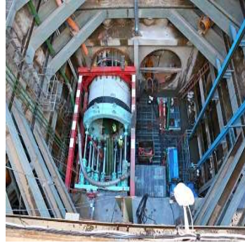
Sewer constructed by pipe jacking method
